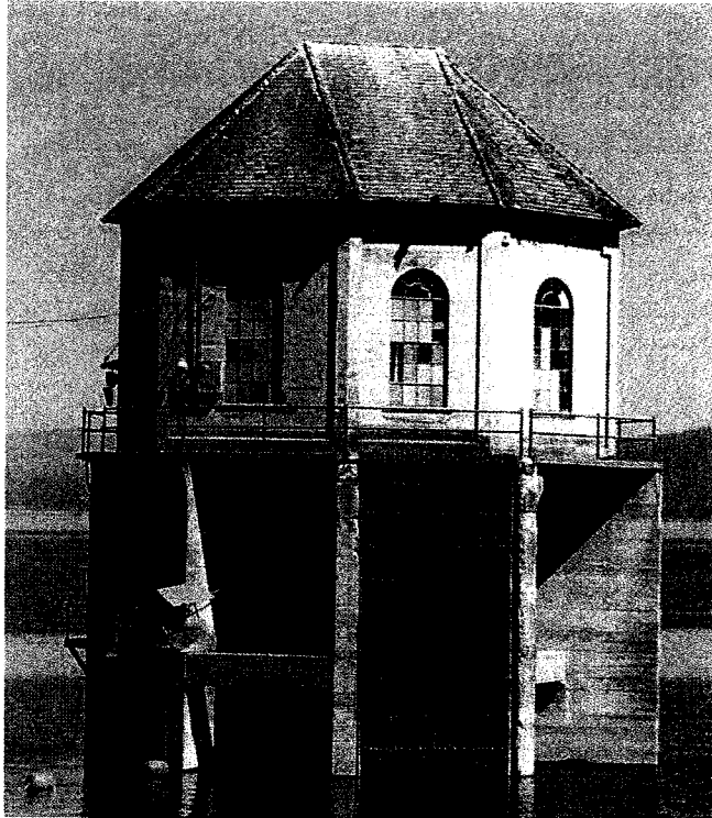
Figure 1: Lake Almanor Intake Tower (August 2006)
